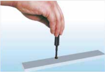
Take out the insert 取出钢丝螺套
